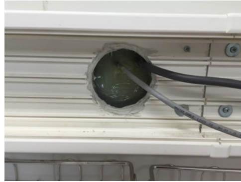
Figure 4: Injected silicone for the sealing of the perforation for electric cables
