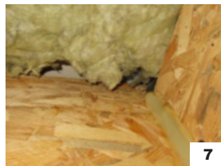
Figure 7: Big gaps between the rock wool insulation and the refurbished wall, leading to air leaks
